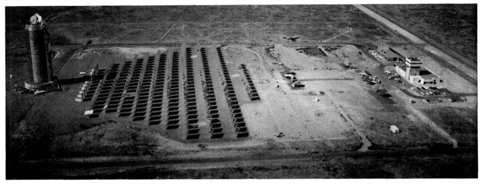
CENTRAL RECEIVER TEST FACILITY was the site of a Molten Salt Electric Experiment, the first US system to use molten salt rather than water to transfer
